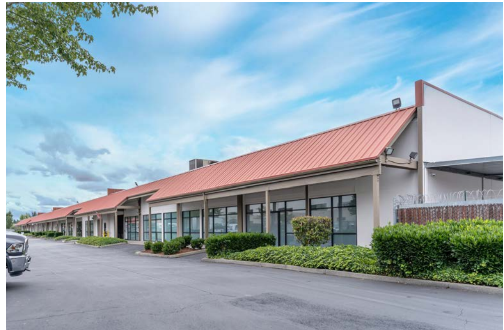
Building D (Industrial)
