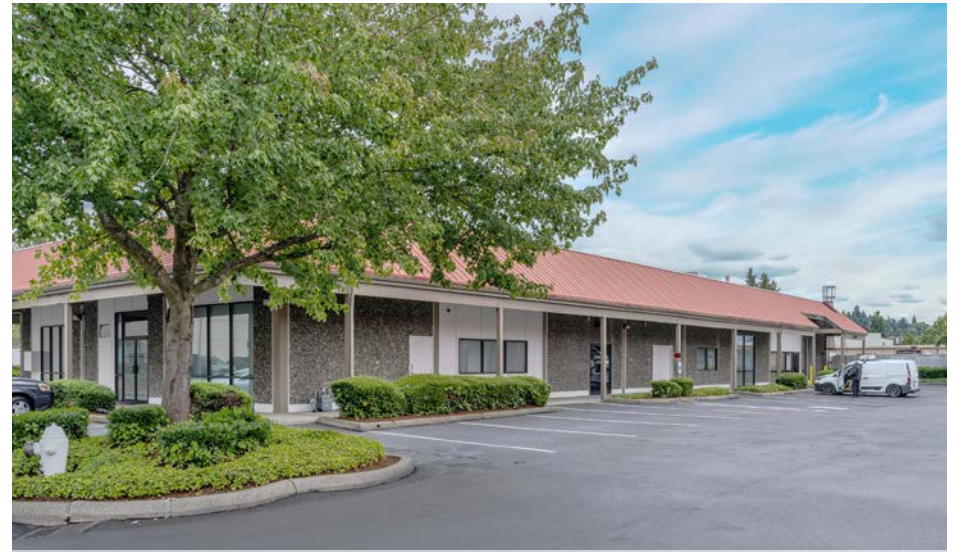
Building B (Flex/Office)
